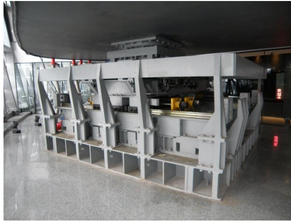
Fig.4 Bi-directional sliding bearing
